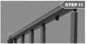
Starting at the angle bracket end, attach each picket one at a time using a slight up and down motion of the top rail as you work your way down.
