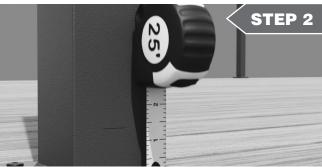
Measure 1-3/8" from the top of the flange and make a pencil mark at that height.
