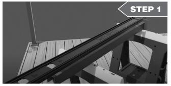
Place the appropriate side of the template against post, based on post width.
