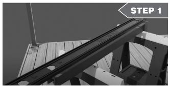
Place the appropriate side of the template against post, based on post width.
